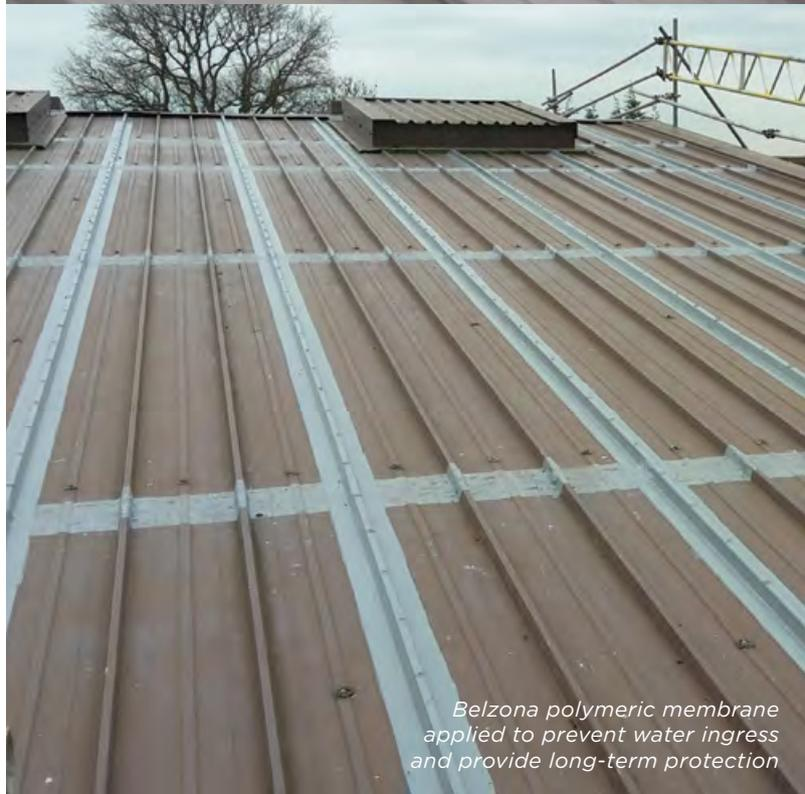
*Belzona polymeric membrane applied to prevent water ingress and provide long-term protection*
