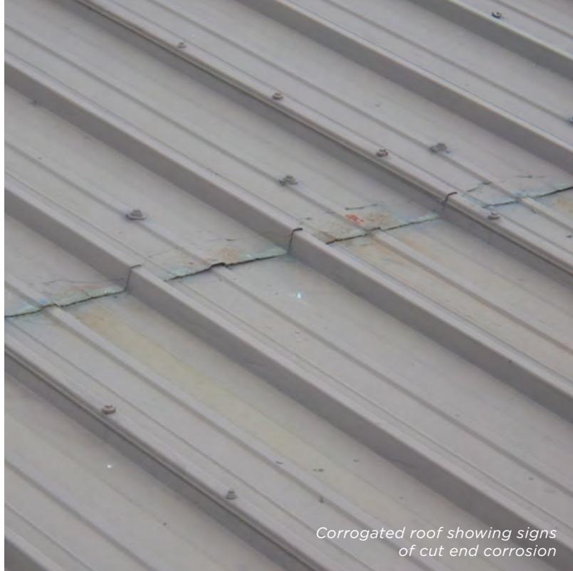
*Corrugated roof showing signs of cut end corrosion*
